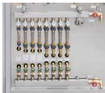
Cooling water distribution
