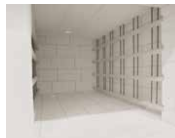
Protection grid in front of heating elements prevent against mechanical damages
